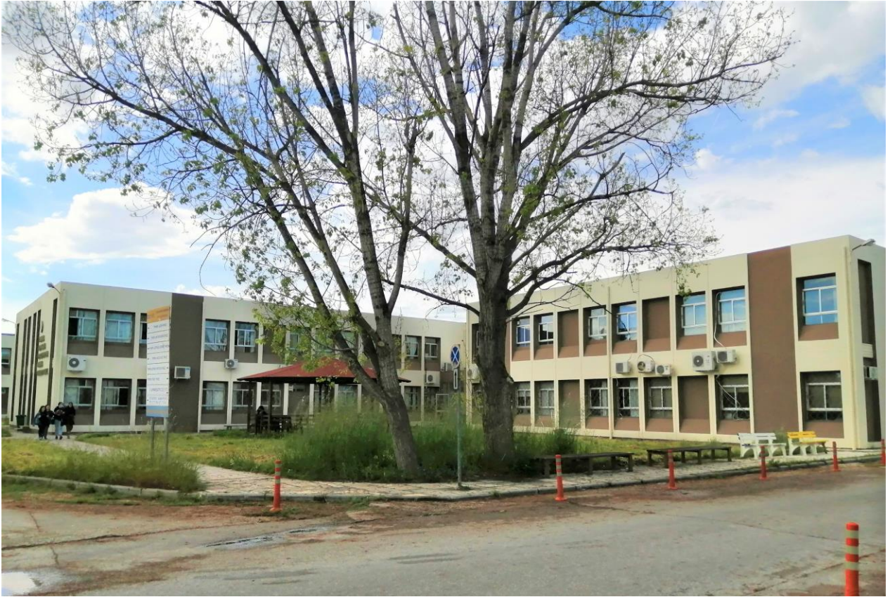
Figure 2. View of the Department's building - BIOMEDICAL SCIENCES -
